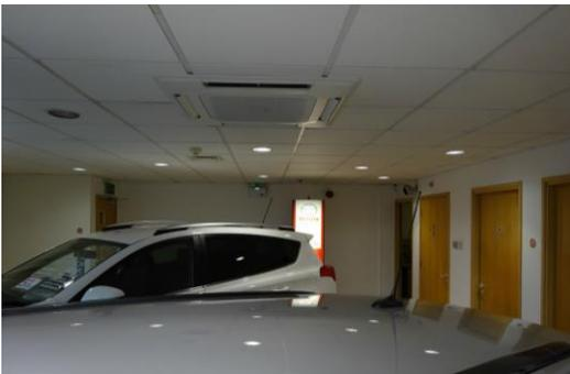
The Hobbs team removed the existing equipment and replaced it with a City Multi Variable Refrigerant Flow (VRF) system.
